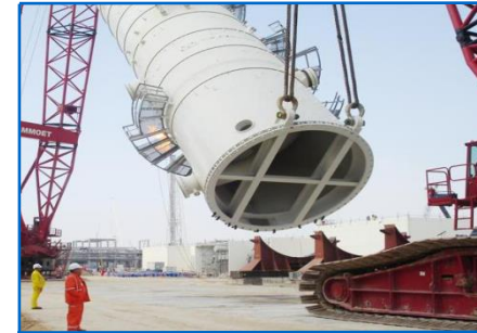
Carbon Capture RECAP Absorber Column Design
