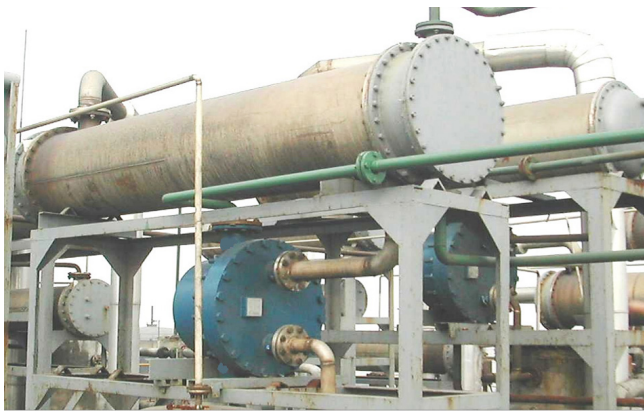
Figure 3. Plate and shell exchanger performing the same duty as shell and tube (with thanks to Robert Broad).
